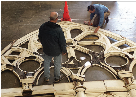
First Congregational Church restoration, Restore Oregon.
